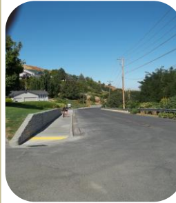
College Street improvements complete! Photos by: Dave Robertson
